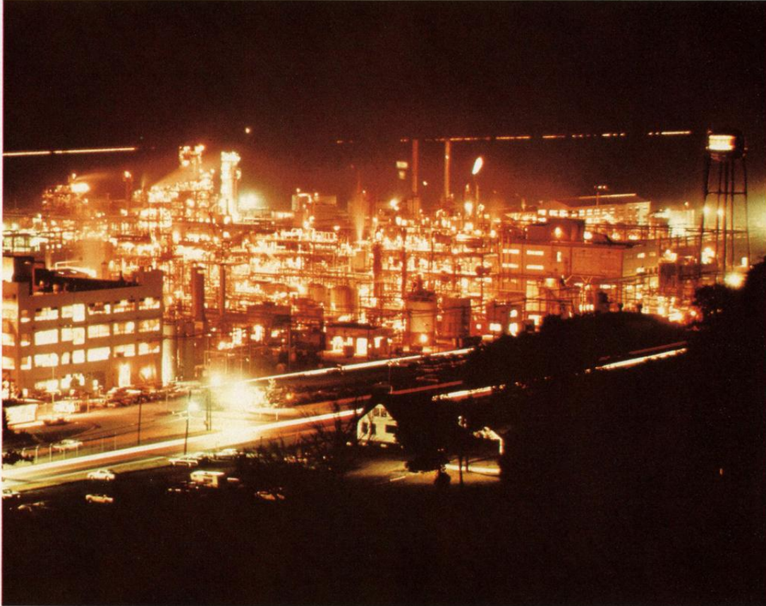
Overseas plants: Mobay, a subsidiary of Bayer, is manufacturing basic materials for plastic production in New Martinsville, USA.
