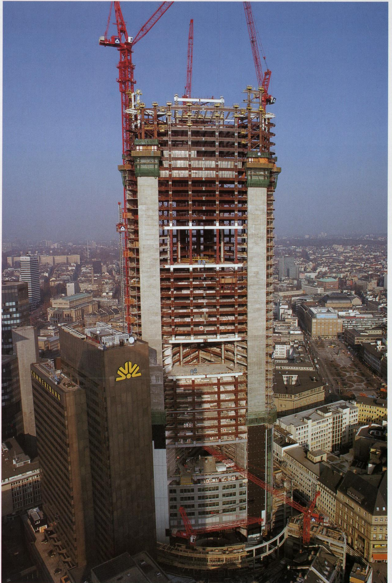
State of progress on January 22, 1996
